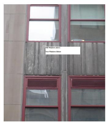
When the Empire State Building had its original windows replaced in 1993, PPG created a customized Duranar coating to match the color of the landmark's original window trim. When 400 more windows were replaced in 2006, PPG was able to match the window color again, even after they had endured more than 13 years of weathering. This was due to the durability and color-fastness of the original Duranar coating, as well as the precision of company's digital color-matching system.
