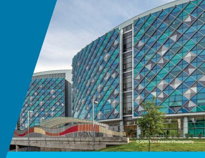
A combination of PPG metal coatings and glass helps to create this bright curtain wall for the exterior façade of the Nemours/DuPont hospital, which has achieved LEED certification at the Silver level.
