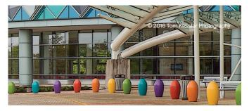
Architects envisioned the signature façade of the hospital to mimic the protective framework of an arbor. The aquablue appearance of Azuria glass is further enhanced by the application of Duranar and Duranar Sunstorm coatings.
