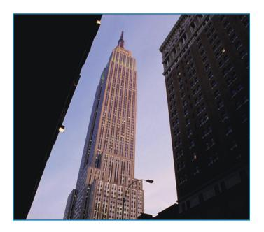
This task was complicated by the initial construction of the building in 1930, which despite its size, was erected very quickly for its time. To speed the construction process, the original architect, William Lamb of Shreve, Lamb & Harmon, ordered the stone columns to be put into place, rough-cut, directly from the quarry without any final cutting or fitting.
