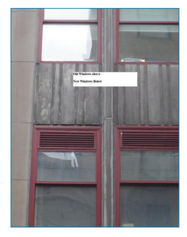
When the Empire State Building had its original windows replaced in 1993, PPG created a customized **Duranar** coating to match the color of the landmark's original window trim. When 400 more windows were replaced in 2006, PPG was able to match the window color again, even after they had endured more than 13 years of weathering. This was due to the durability and color-fastness of the original **Duranar** coating as well as the precision of company's digital color-matching system.
