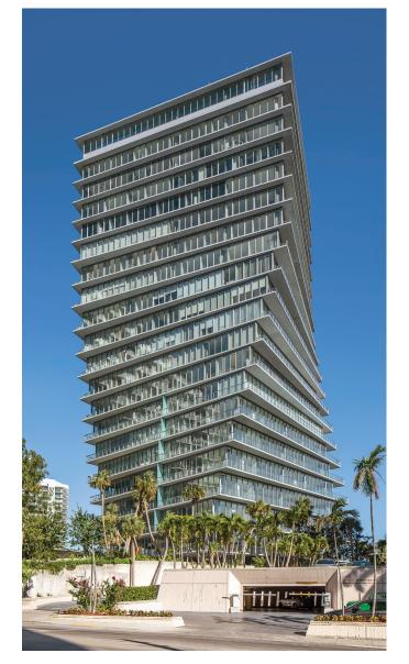
Tecnoglass selected *Duranar* coatings for the Grove at Grand Bay because they offer the proven seacoast corrosion performance required for projects in humid, salt-air environments.
