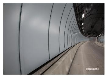
The 4,000 solid aluminum plate panels lining the tunnel were painted with Duranar XL Crystal Blue coatings, while the lattice work was coated with durable Duracron coatings.
