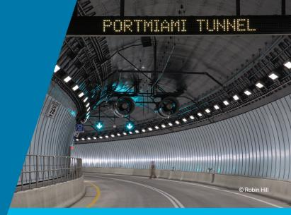
Duranar XL and Duracron coatings by PPG were specified for use in the PortMiami Tunnel, South Florida's newest landmark, because they combine bright color with exceptional resistance to abrasion, salt, humidity, car exhaust and fading.
