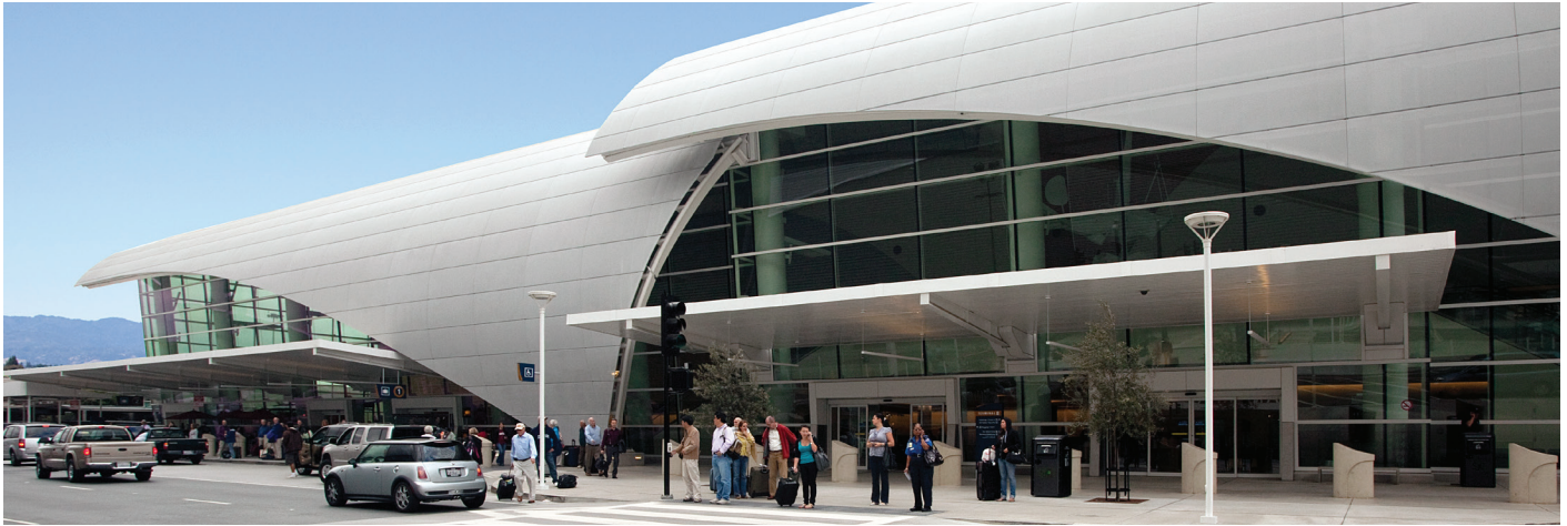
Duranar powder coatings in Regal White coat the perforated panels that envelop San Jose International Airport's Terminal B.
