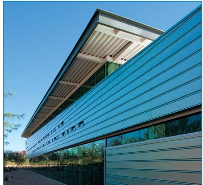
*The Appaloosa Branch Library in Scottsdale, Ariz., features Solarban 60/Atlantica glass and metal panels with color-shifting Duramar VARI-Cool coatings to control energy costs and help the building blend into its desert setting.*
