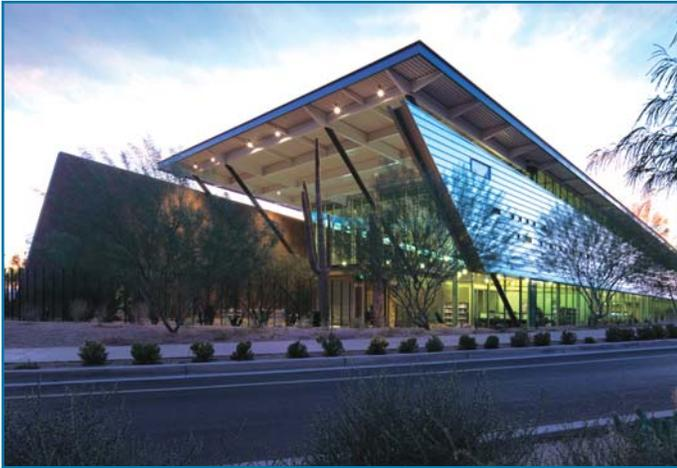
*Duranar VARI-Cool* coatings on the Appaloosa Branch Library shift from dark green to silver to mauve, depending on light conditions and viewing angle.
