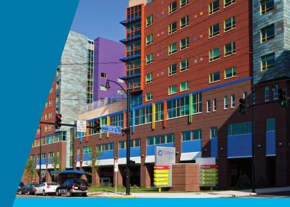
Coraflon and Duranar fluoropolymer coatings were specified for their low-maintenance requirements, increased durability and color retention. The Coraflon coating colors shown here provide bright and vivid colors on the exterior of Children's Hospital of Pittsburgh of UPMC.
